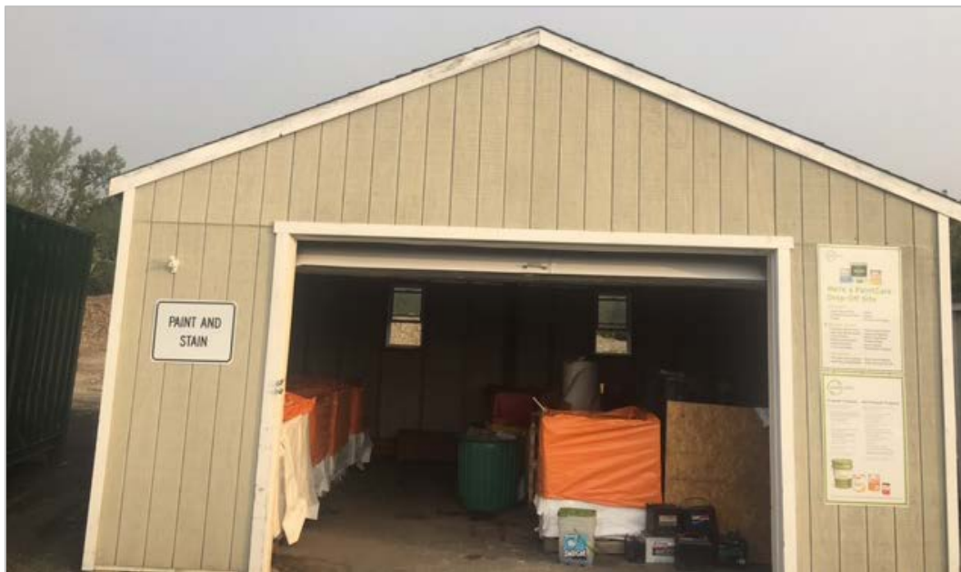
Paint Bins and Signage at the Watertown Transfer Station
